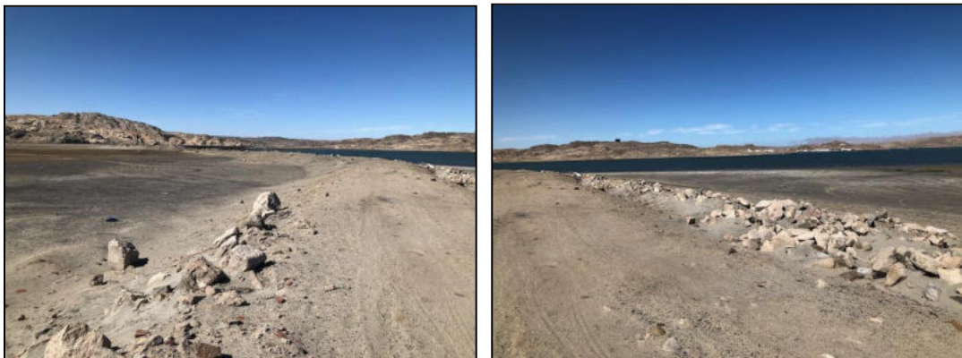
Figure 11: Gravel wall which prevents the sea from flooding Erven VX and VIX
