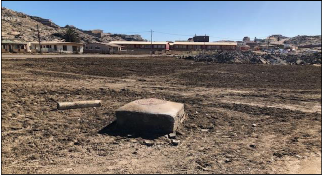
Figure 14: Sewage connection on site
