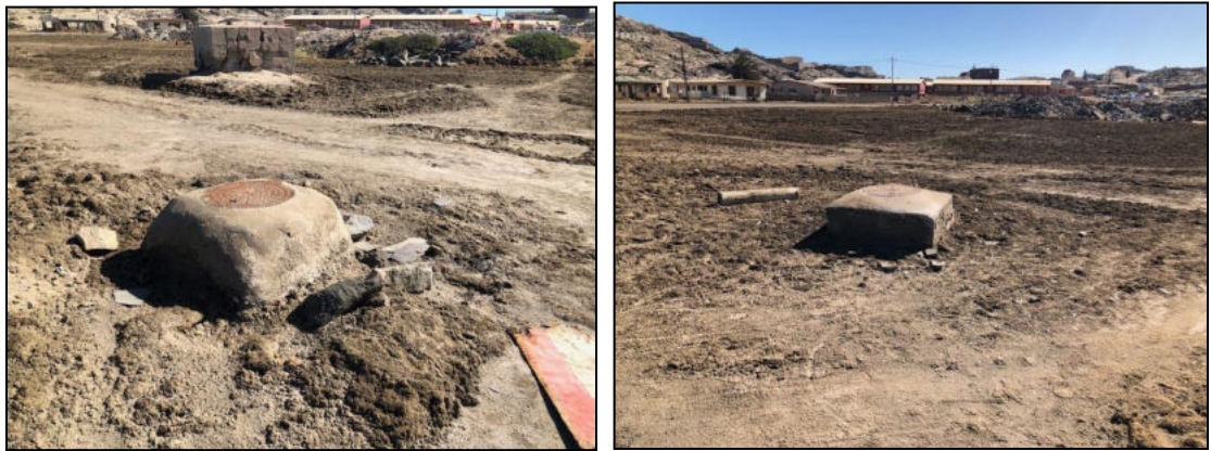
Figure 15: Photo showing manholes of the sewer line
