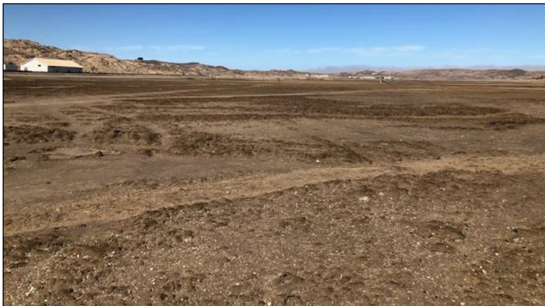
Figure 4: Image of the Project Site area (1)
