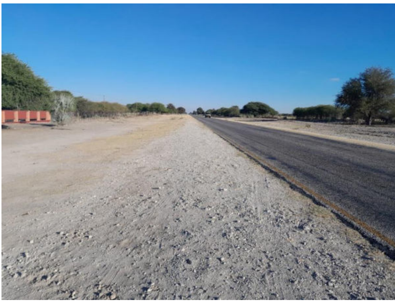
Figure 10: B1 main road-access road to the project area
