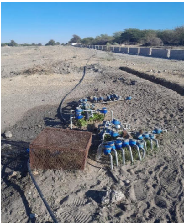
Figure 11: Portable water connection made to the existing bulk water services
