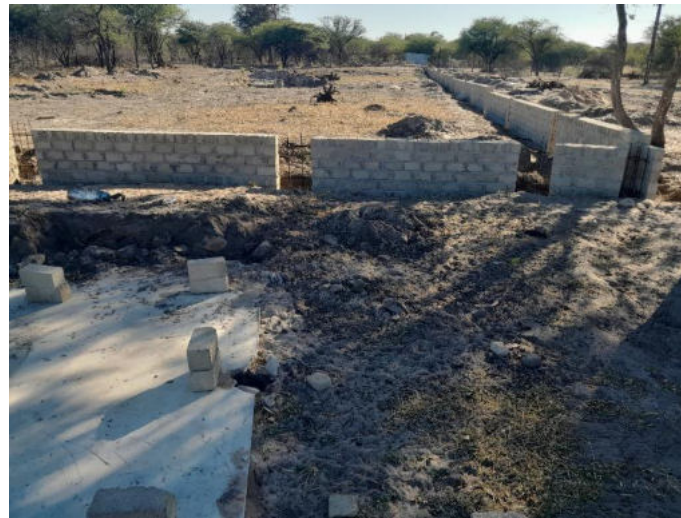
Figure 1: On-site project existing constructed boundary wall
