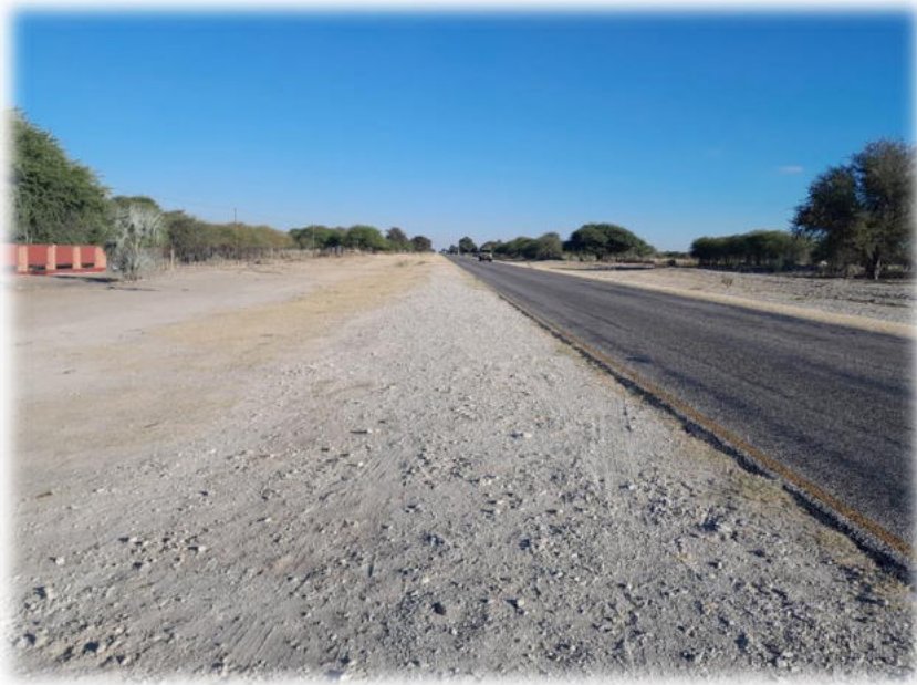
Figure 7: B1 Tsumeb-Omuthiya tarred road (Access Road to the project site on the left)
