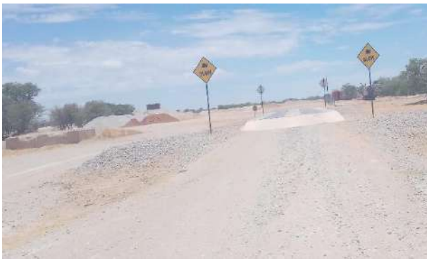
Figure 7: Weighbridge seen from entry side
