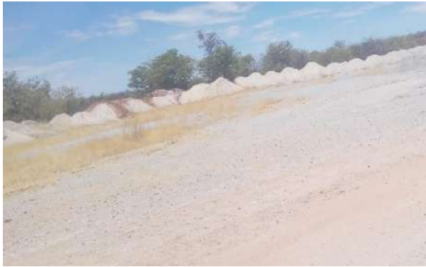
Figure 5: Crusher fines used as berms along C41
