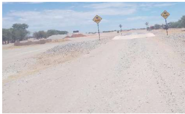
Figure 34: Internal routes & signage at the weighbridge
