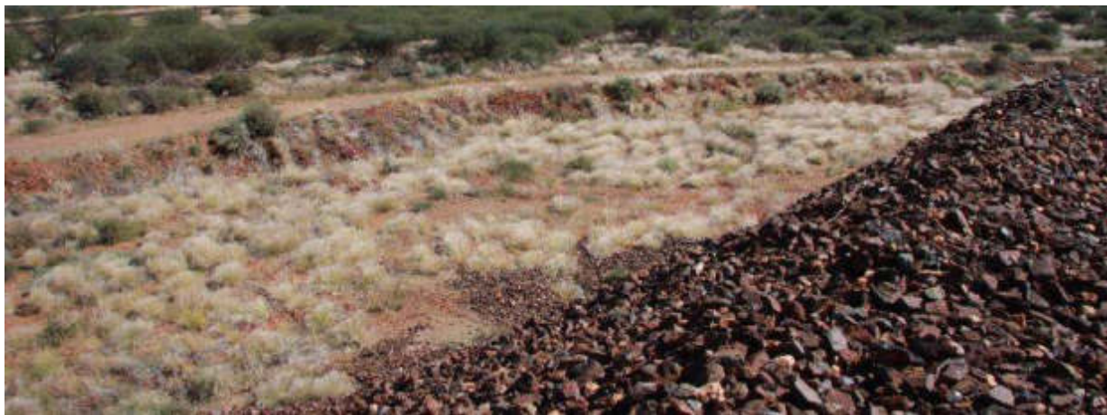
Figure 9: An earth berm below the excavated area and stockpiles made to contain the rainfall runoff on the site
