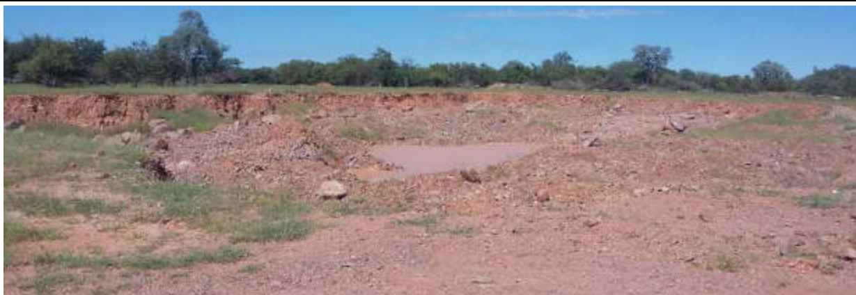
Figure 5: Shallow Excavated Trenches – photo taken March 2017. Note pooling of rainfall water in the trench
