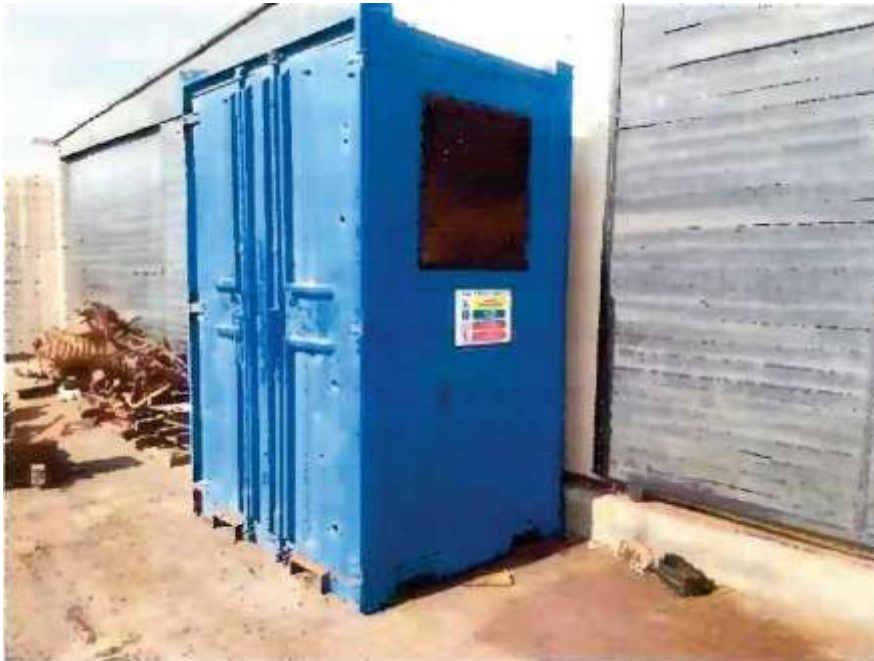
Figure 9. Compressed Gas Storage
