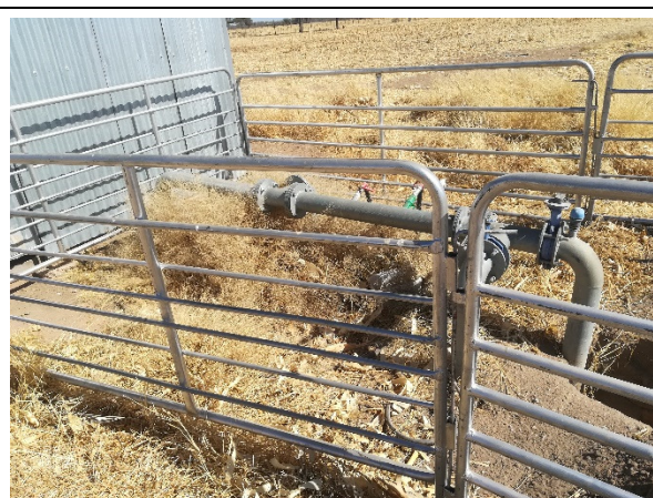
Photo 4-14. Guarded borehole installation
