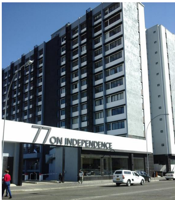
Precautionary measures... The residential and retail complex on Independence Avenue where Namibia's 33rd Covid-19 case was traced to. Photo: Contributed
