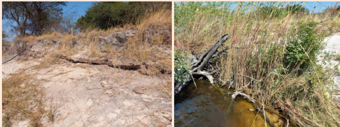
Figure 7: Reeds were planted (~June 2022) in an attempt to protect the river bank (Source: J. Steyn, 01 August 2023).
