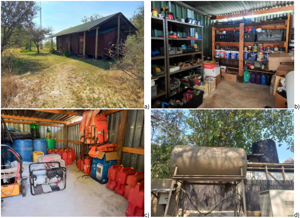
Figure 3: Pictures showing: a) the Assistant Manager's house; b) workshop / tool-shed; c) fuel store; and d) fuel tank and generator (to the right) (Source: J. Steyn, 01 August 2023).
