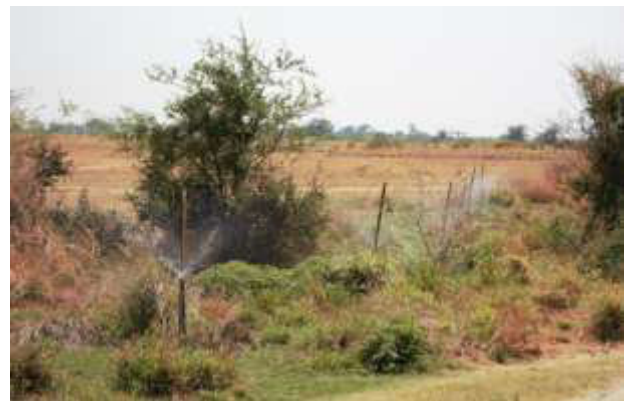
Figure 9 Final effluent release through sprinklers
