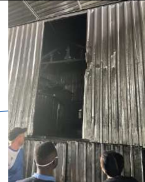
Crusher closed off to minimize dust emissions.
