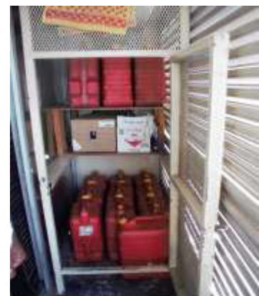
Figure 7 Storerooms for fuels
