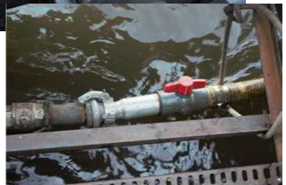
Figure 6 Pumping out of effluent from the houseboat
