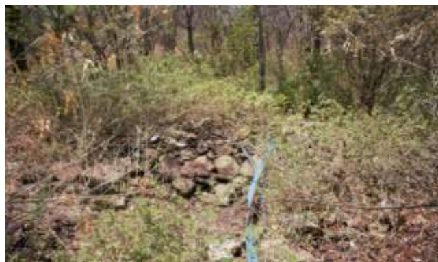
Figure 12 Discharging of Laundry water
