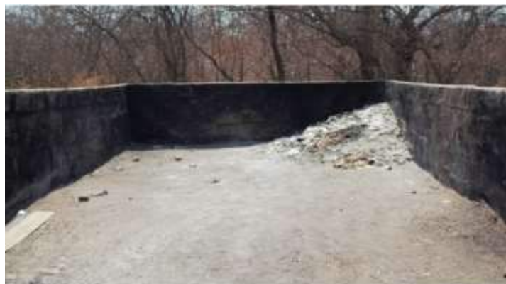
Figure 9 Incineration area for combustible waste
