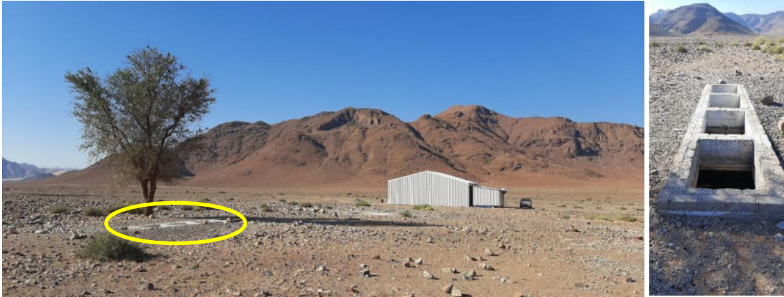
Figure 9: Structure to be removed / filled with sand so as to not pose a hazard to humans and/or animals (Source: L Maartens, July 2023).
