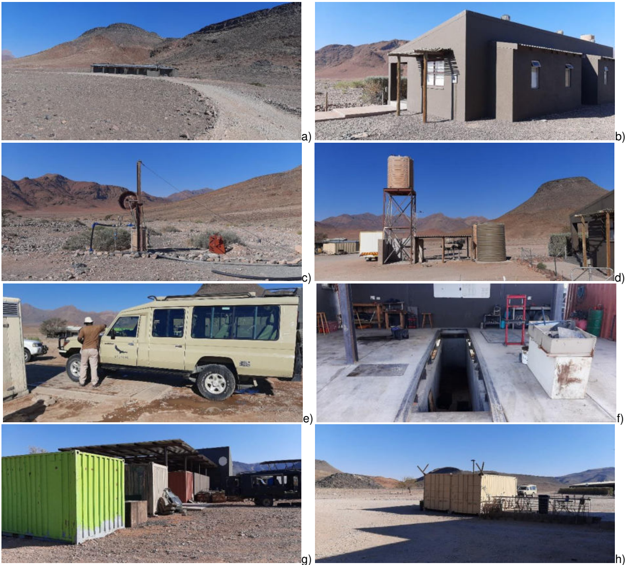
Figure 8: Pictures showing: a) and b) Staff Village accommodation; c) borehole infrastructure; d) three 10,000 litre water storage tanks; e) wash bay; f) two workshops and a service pit; g) three storage containers; and h) additional two storage containers (Source: L Maartens, July 2023).
