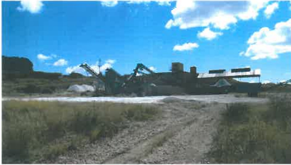
Figure 3: Peralin crusher and screen plant
