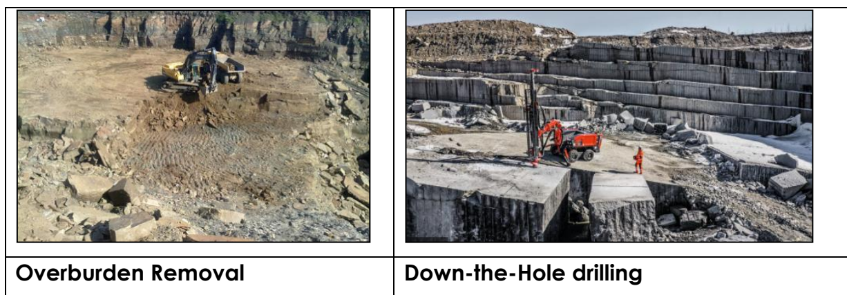
Figure 2: An example of some of the techniques to employed in this exploration project.
