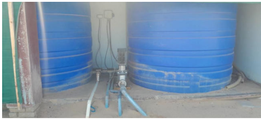
Figure 12: Sea-water pump station and the x3 10,000 litre water reserve tanks
