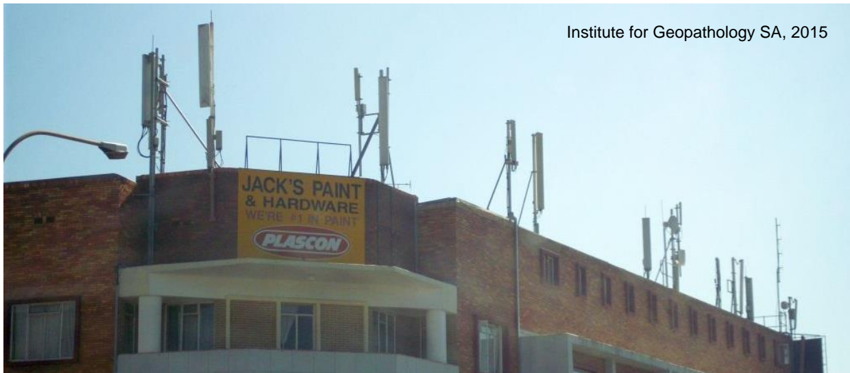
Figure 5-9: Example roof top BTS
