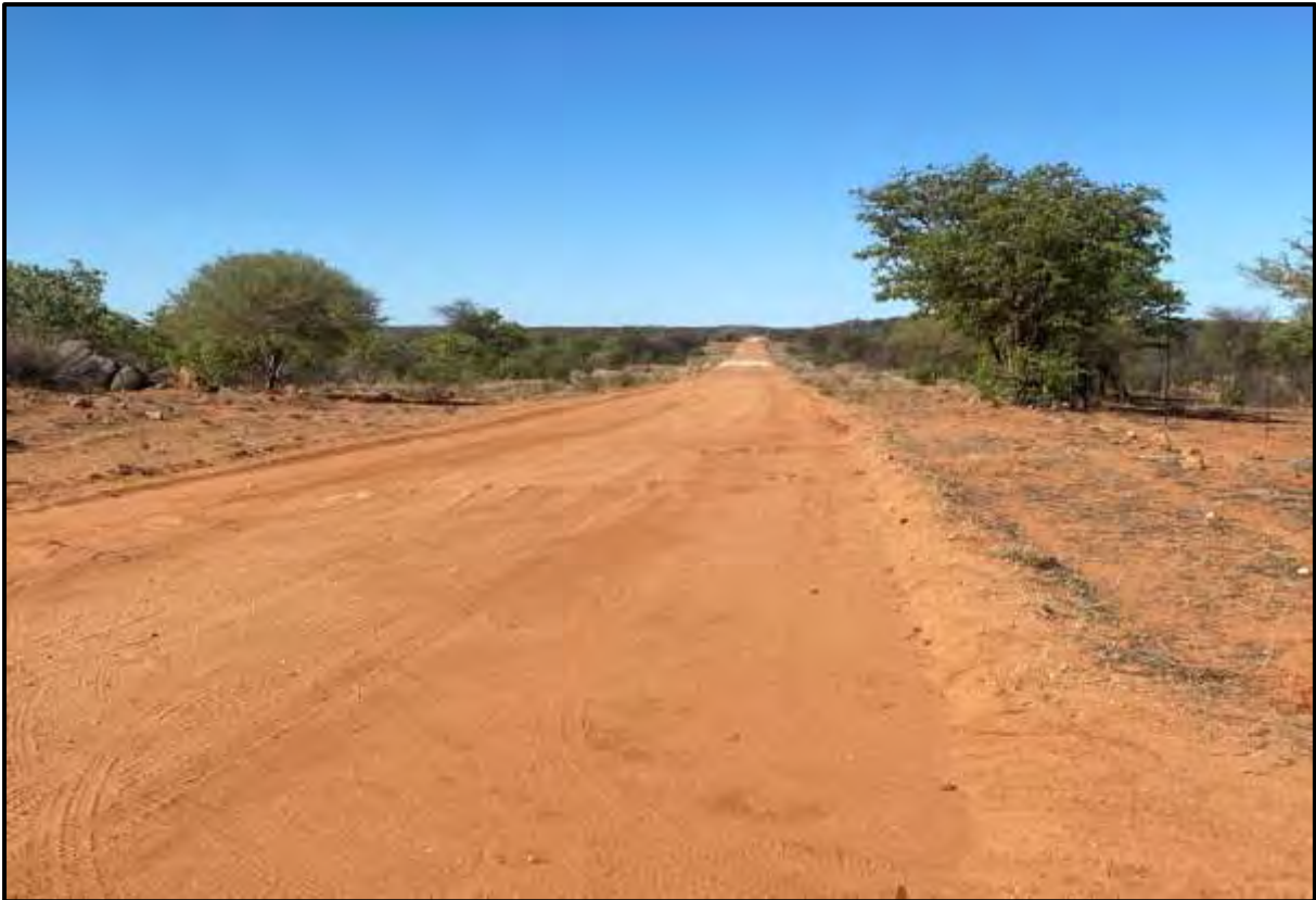
Figure 3-3: Well-maintained D2666, Gravel/graded Road within the EPL area.
