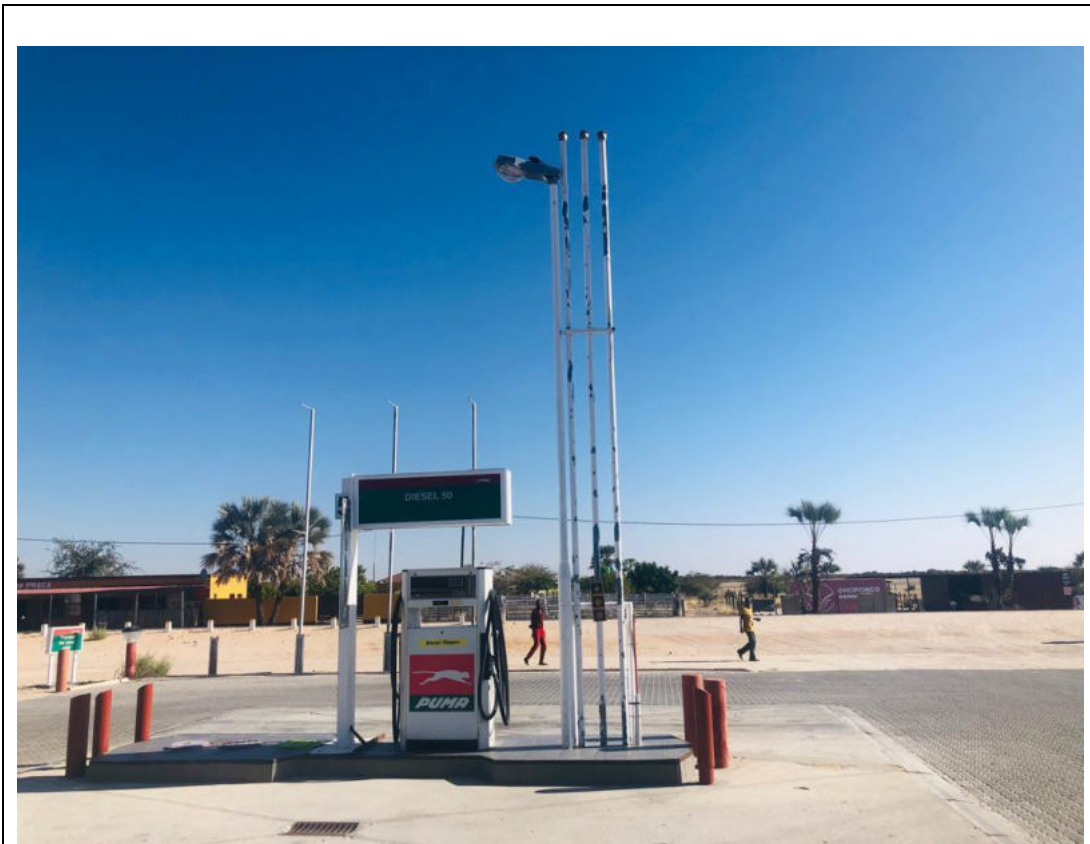
Image 1: Vent pipes have been installed on site (3m) to release vapors above the immediate atmosphere to enhance pollution attenuation.
