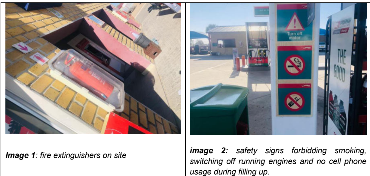
Figure 5: fire and safety control measures currently on site
