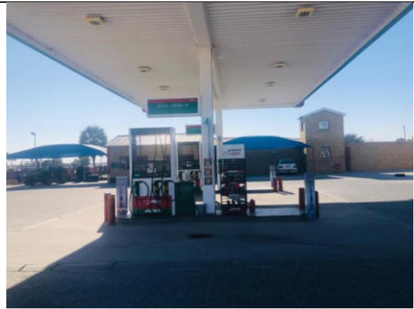
Image 2: A concrete slab for surface spills containment.
