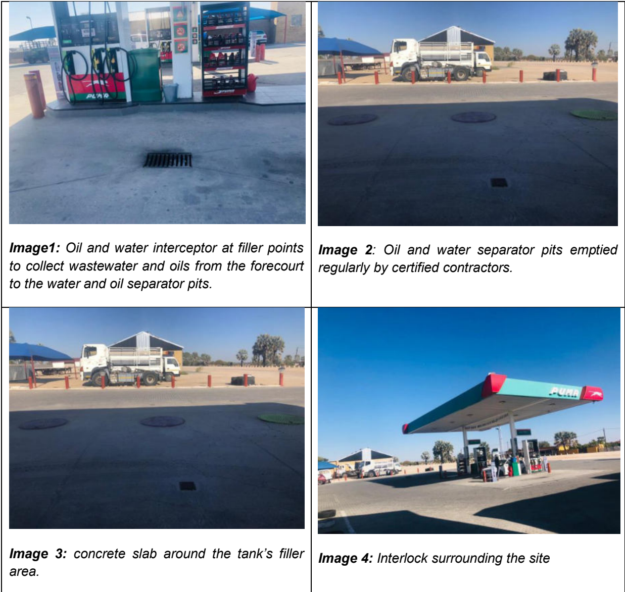
Figure 2: underground pollution control measures currently on site
