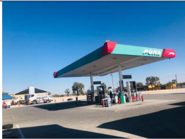
Image 1: A canopy installed on site
