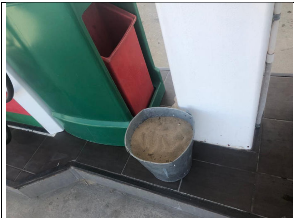
Image 1: sand buckets on site
