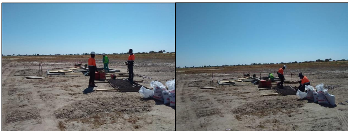
Figure 4: Some of the construction workers on site
