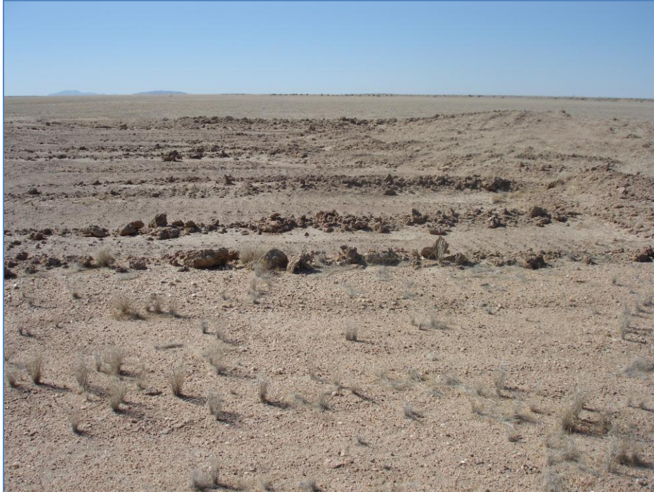
Figure 53. Visible damage of bulk sample pits by previous exploration company in the Aussinanis EPL.
