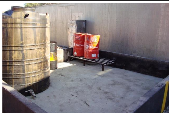
Photo 4-4. Used oil storage in bund area
