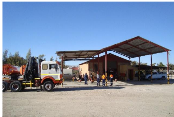
Photo 4-2. Infrastructure on site
