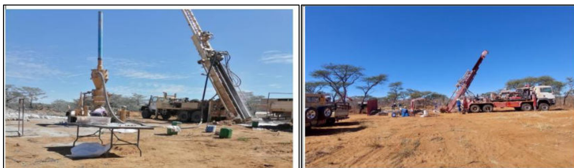
Figure 2-3: A drill rig on an EPL in the Omaheke Region (Resilient Environmental Solutions, 2022)
