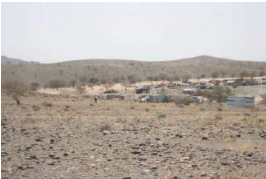
Figure 56. The drainage line running through the northeastern boundary of the ML134 is severely affected by various anthropogenic activities, mainly informal settlement, with most of the trees being felled for fuel.
