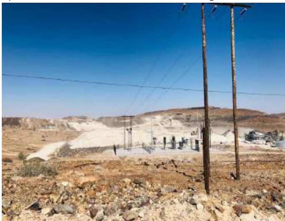
Figure 21 - Main power supply off-take (Source: ECC, 2021)
