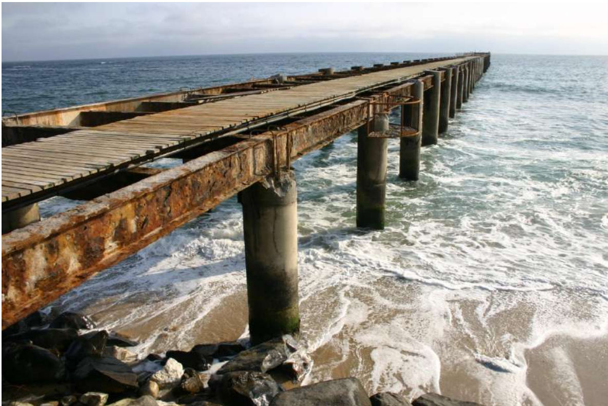
The steel jetty after restoration in 1998
