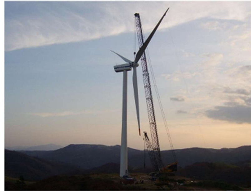
Figure 6: Wind Turbine Installation
