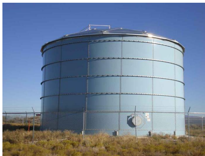
Sample Municipal Potable Water Storage Tanks – Courtesy Erongo Consulting Group, 2020
