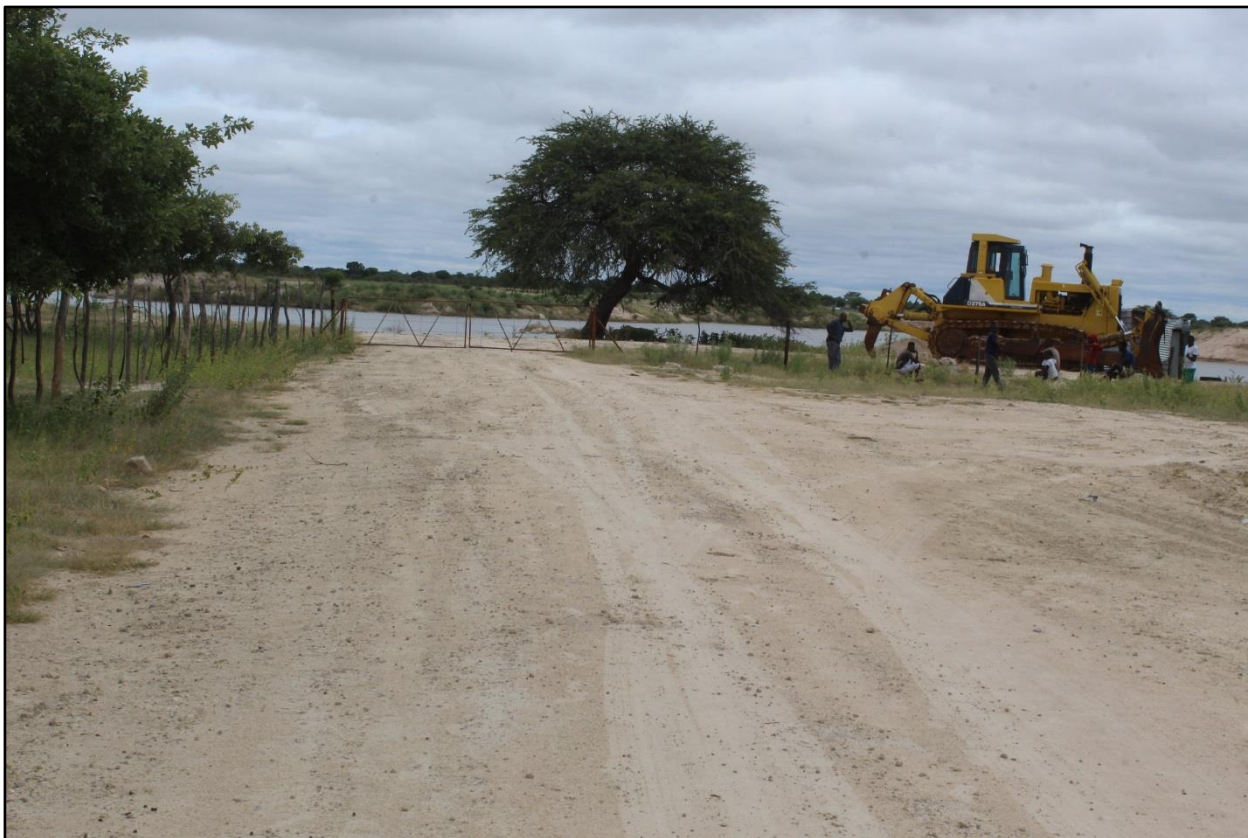
Figure 4: A set of the sand mining and loading machinery on site
