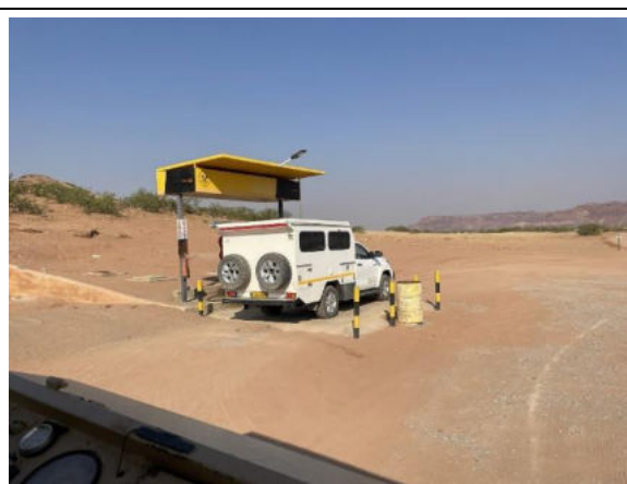
Photo 3-8 Fuel retail facility
