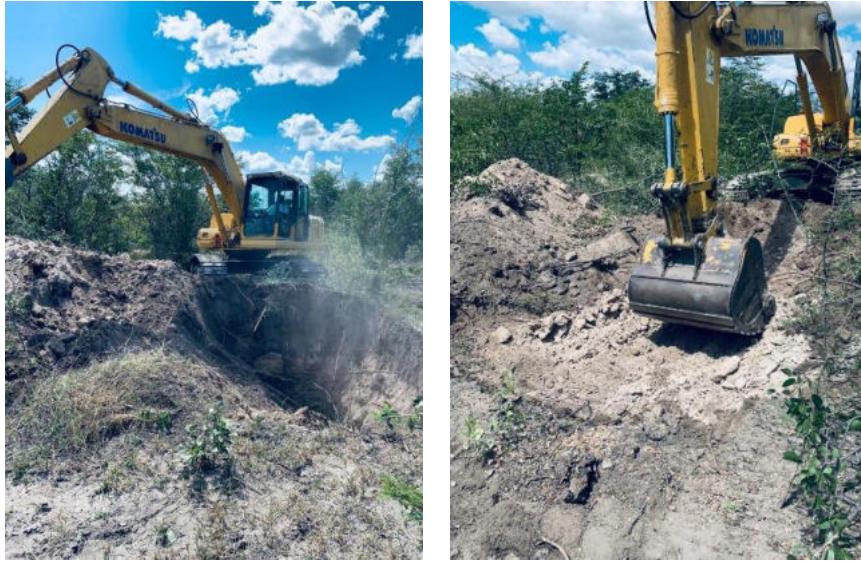
Figure 6: Machinery that is used to dig during borrow pit investigations.
