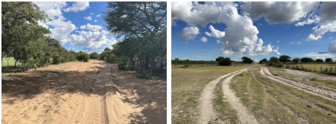
Figure 1: The current condition of the earth track sections is either thick loose sand or pools of water when it rains.
