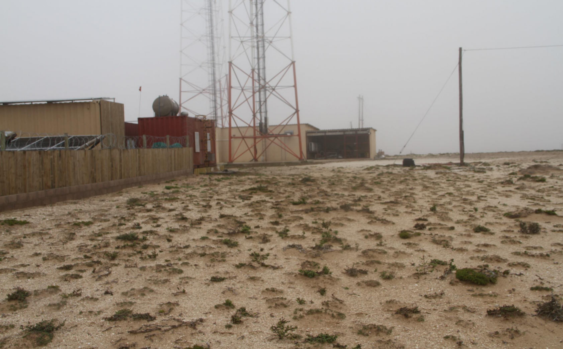
Plate 1.3: Existing supporting infrastructure Kerbehuk line of sight communication station.
