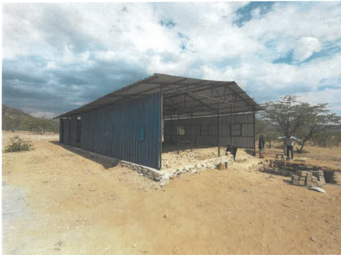
Figure 11: The storage warehouse under construction near the proposed mining sites (HEEC, 2023).
