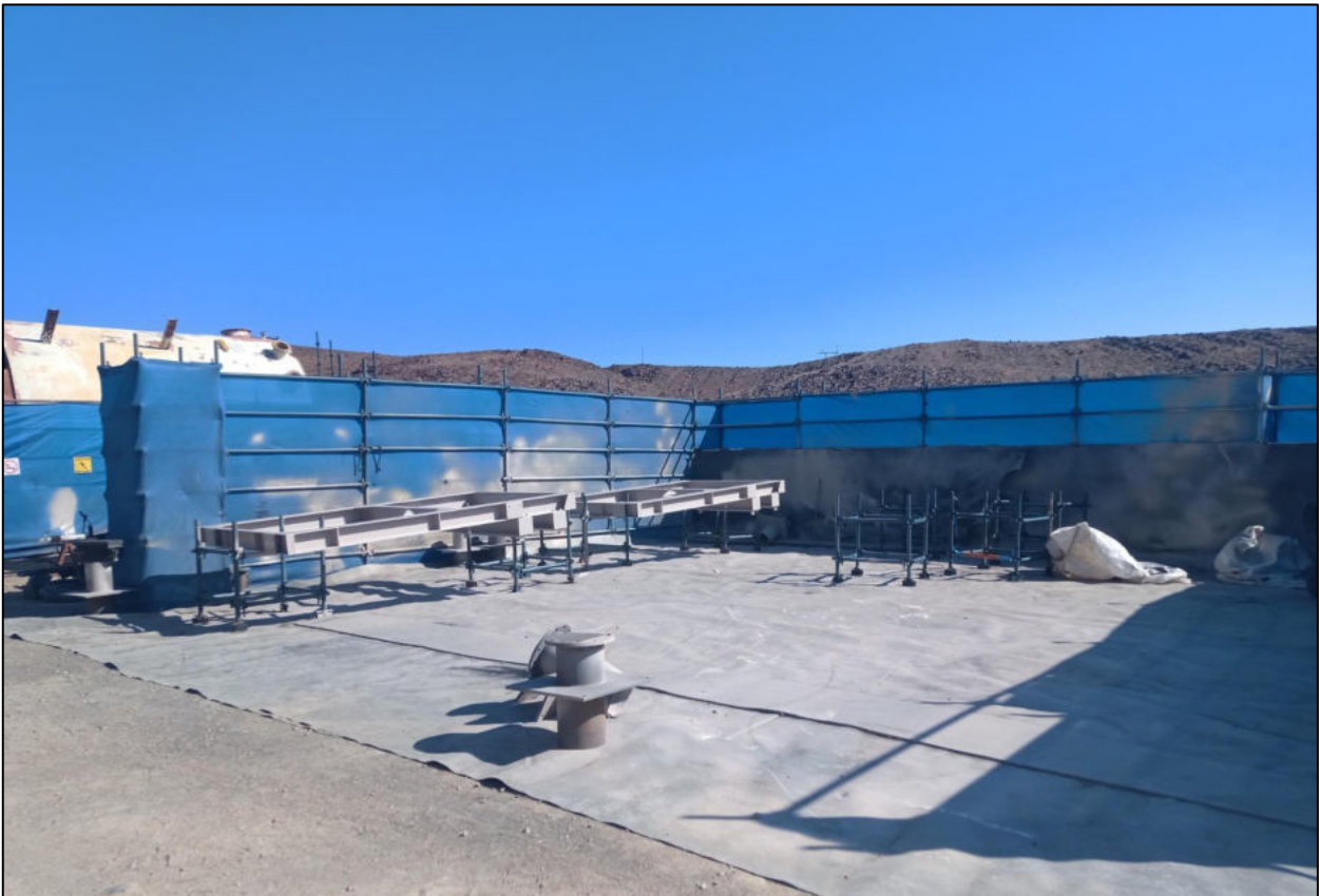
Photo 2: Painting area with lining to prevent spillage
