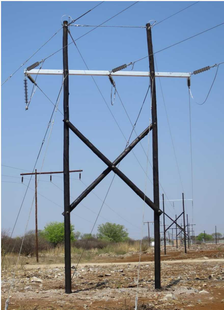
Plate 2.2: Example of the 66kV wooden structure with steel crossarm (Source: Transmission Consulting Services (TCS), 2020).
