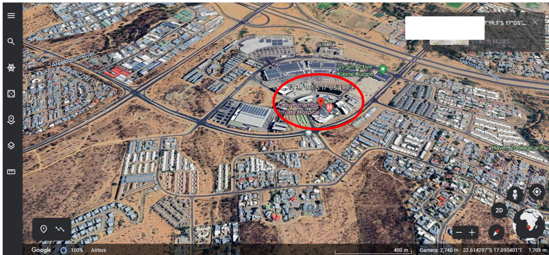
Location of Lady Pohamba Private Hospital where the STERILWAVE Apparatus/Equipment is located (in the Premises Buildings)
