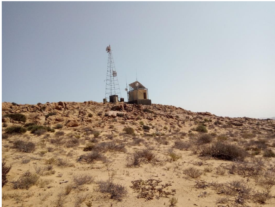
Figure 4: Existing Tower and Radio Receiver adjacent to the proposed site.
