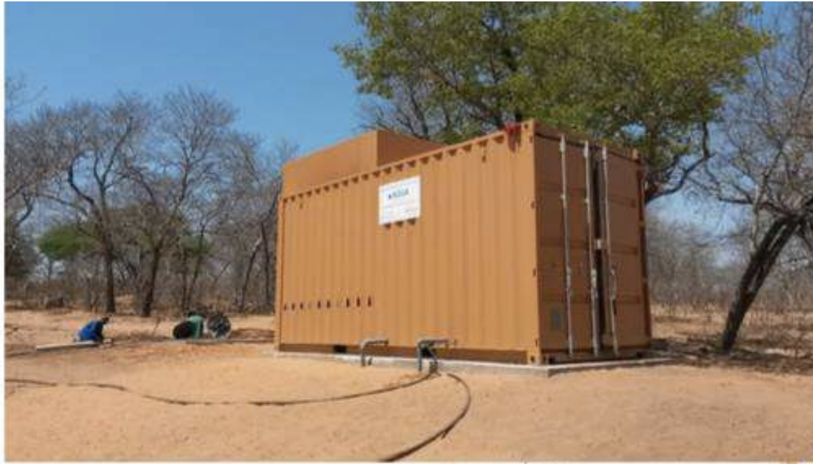
FIGURE 3 - TYPICAL CONTAINERISED SEWERAGE (TRICKLING) TREATMENT PLANT.
