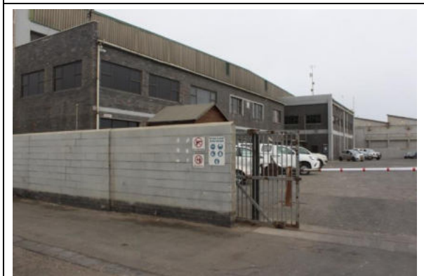
Photo 4-4 Main entrance with security
