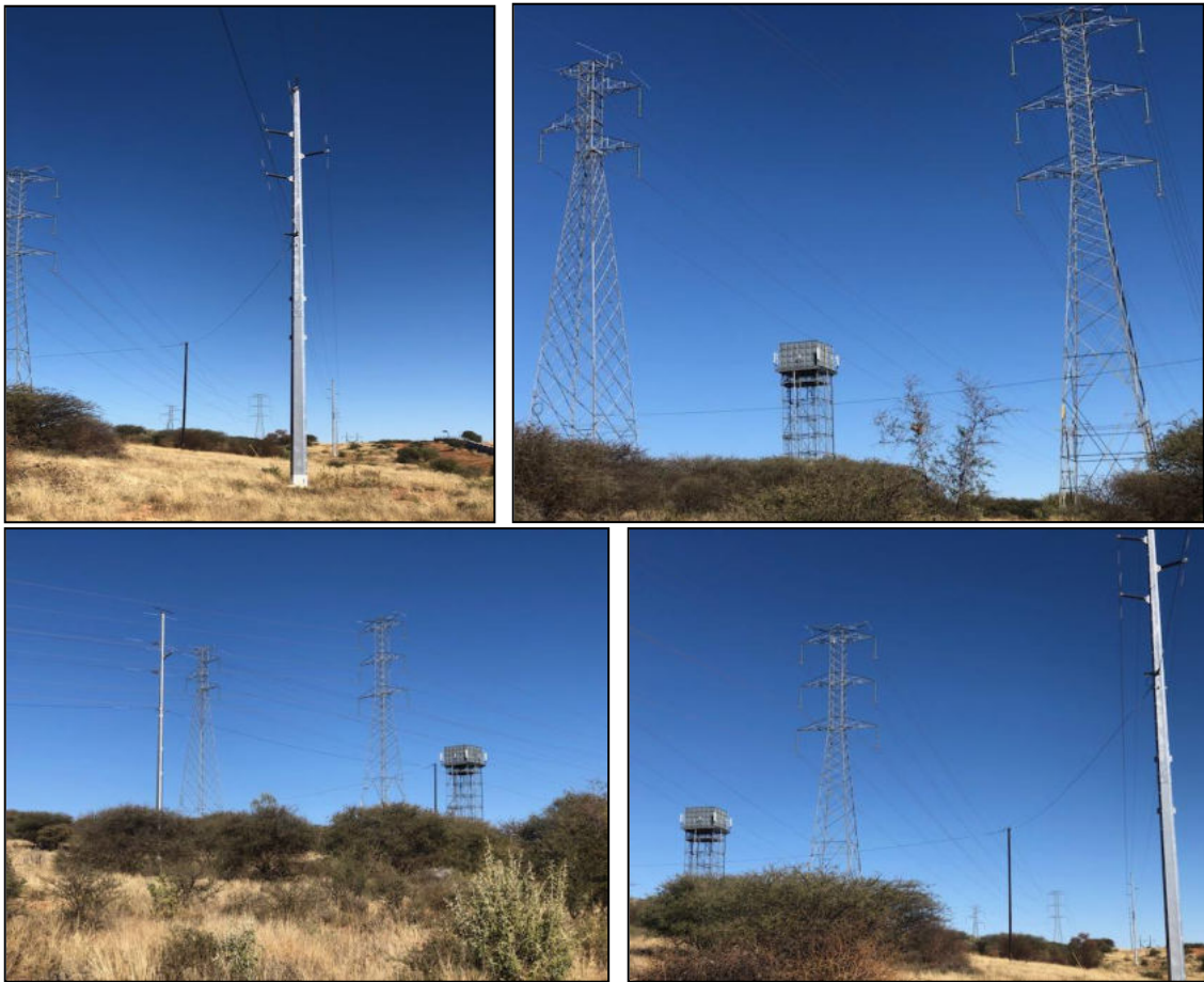
Figure 6: Power line structures and elevated water tank located along the southern boundary of Erf 1
