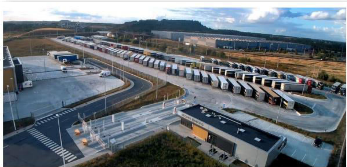
Figure 19: Illustrative envisaged design of the proposed Walvis Bay truck port development (also see page 27 & 28)
