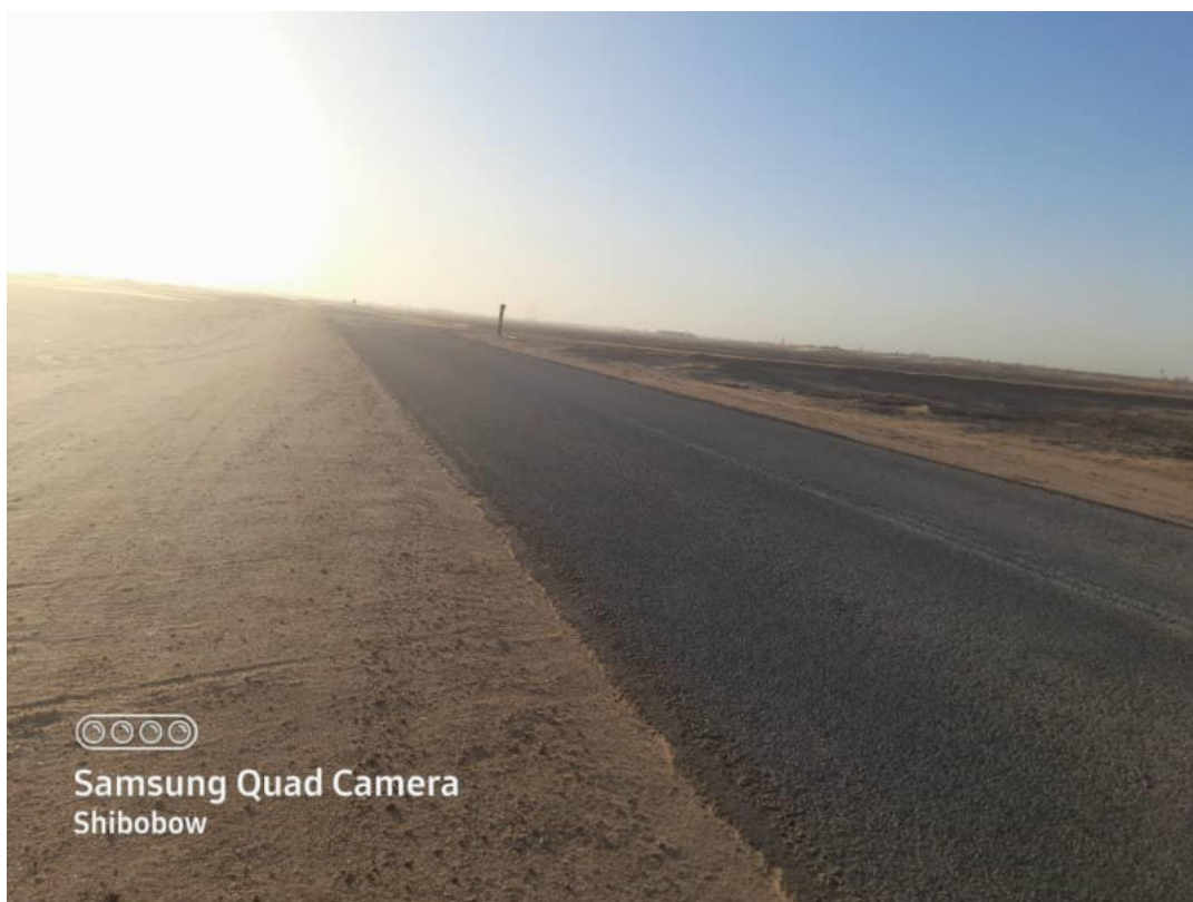
Figure 3: C14 Access-road to the project site
