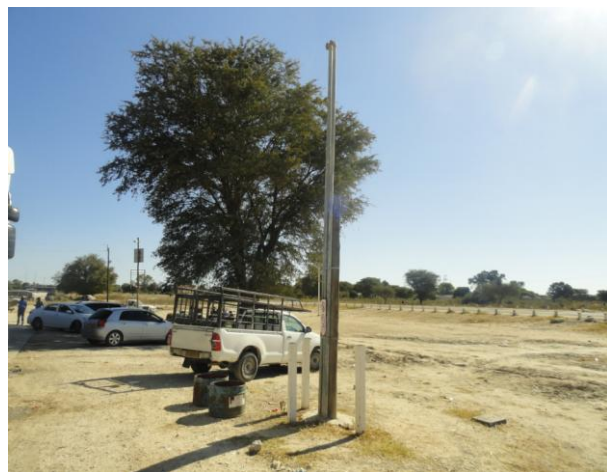
Photo 4. Existing venting pipes
