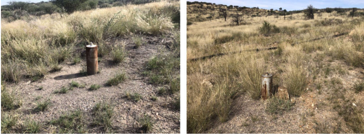
FIGURE 11: UNLOCKED MONITORING BOREHOLES
