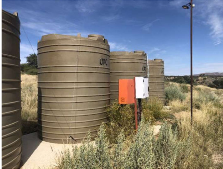
FIGURE 7: THE PLASTIC TANKS TO WHICH THE WATER IS PUMPED FOR DISTRIBUTION ONSITE
