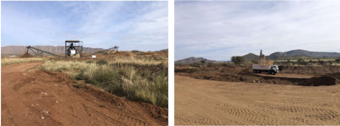
FIGURE 15: DUST GENERATED BY SCREENING, LOADING AND HAULING
