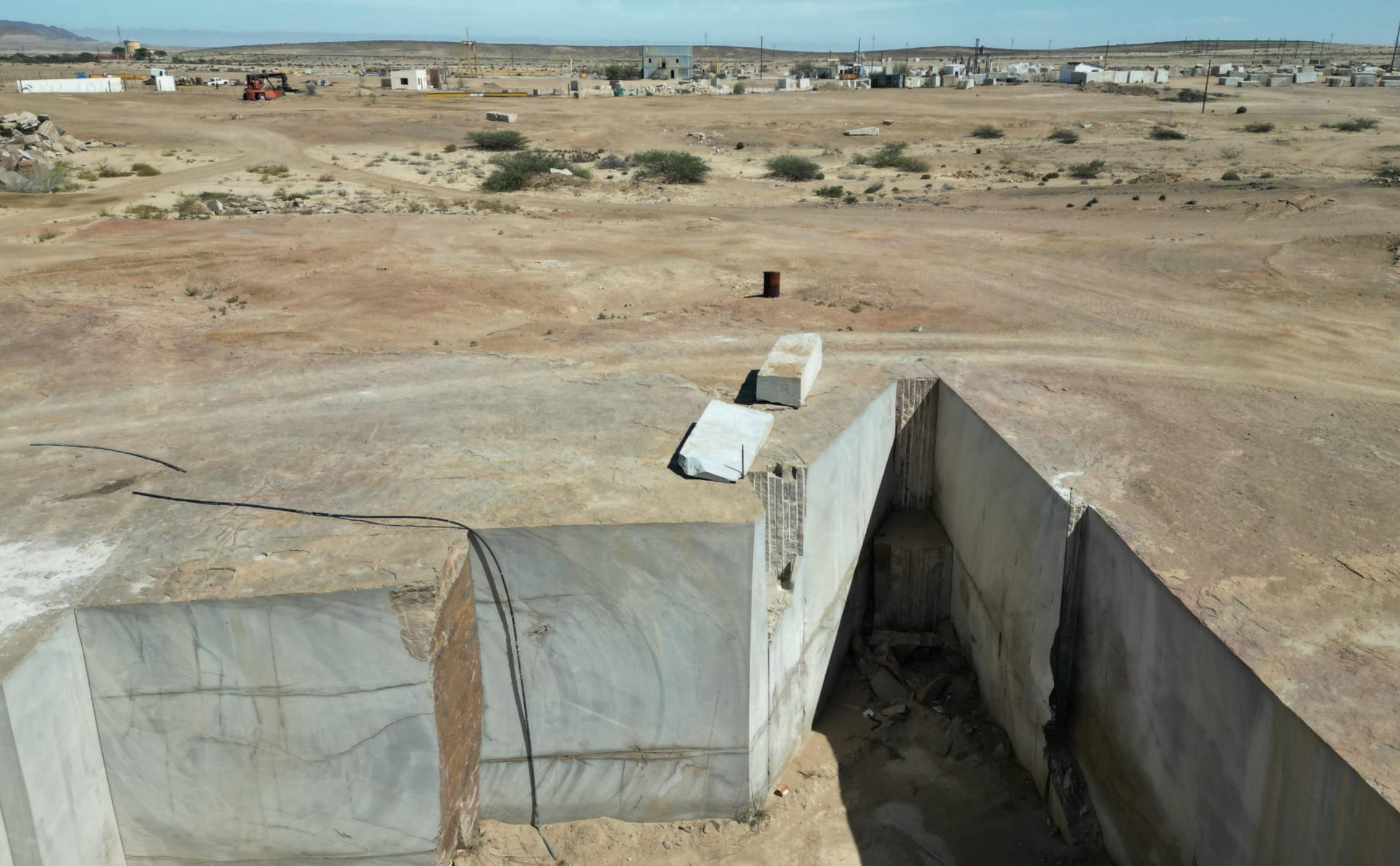
Plate 2.3: Drone image showing the eastern view of the working / extraction face and extracted materials at a granite quarry in the ML No. 120 with the workshop area in the background.
