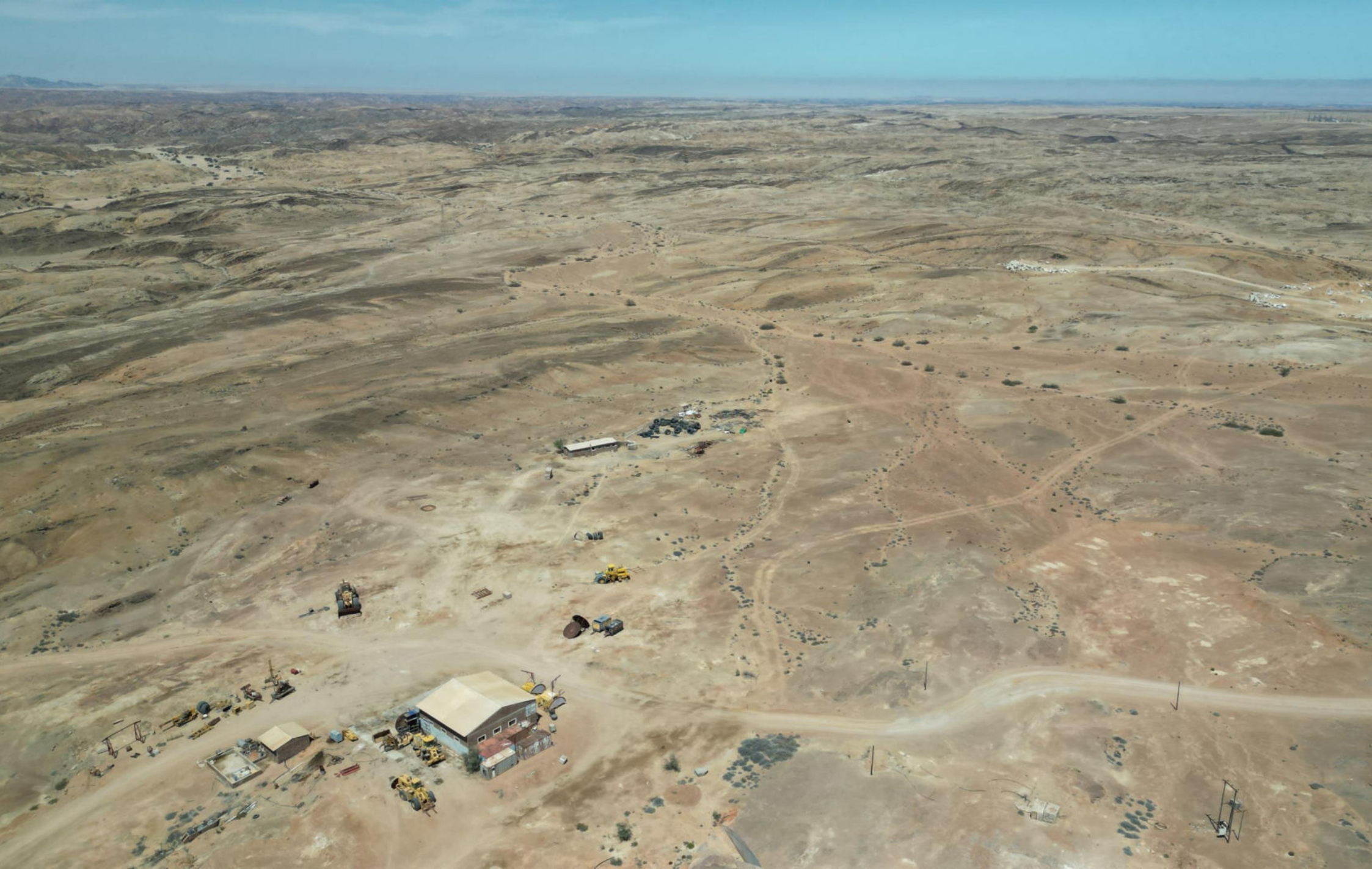
Plate 1.3: Drone image view to the southwest working face of one of the quarries found in ML No. 121 with the workshop in the background.
