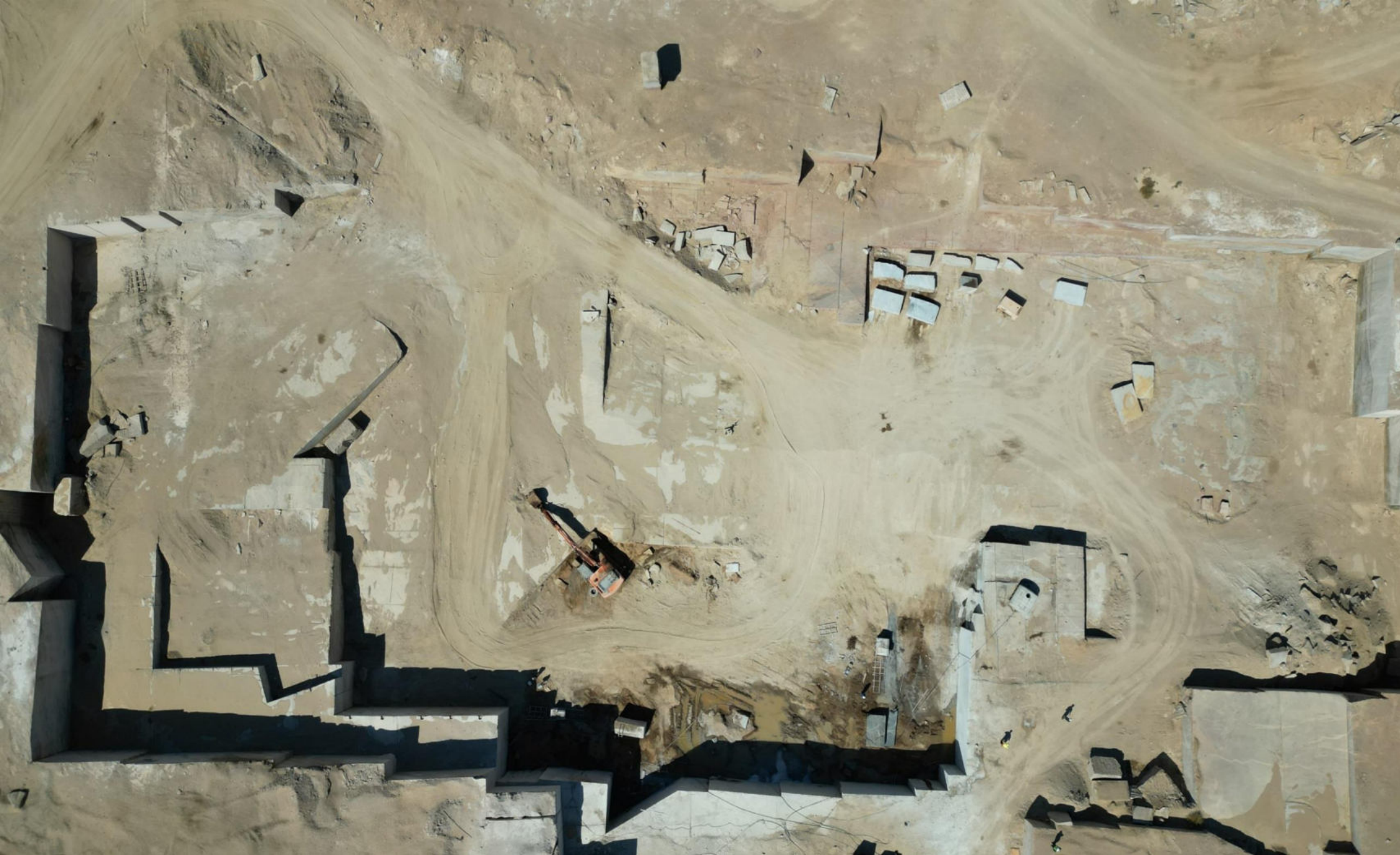
Plate 2.1: Overhead drone image view of the granite in the ML No. 120 showing the granite blocks extraction / operational faces.
