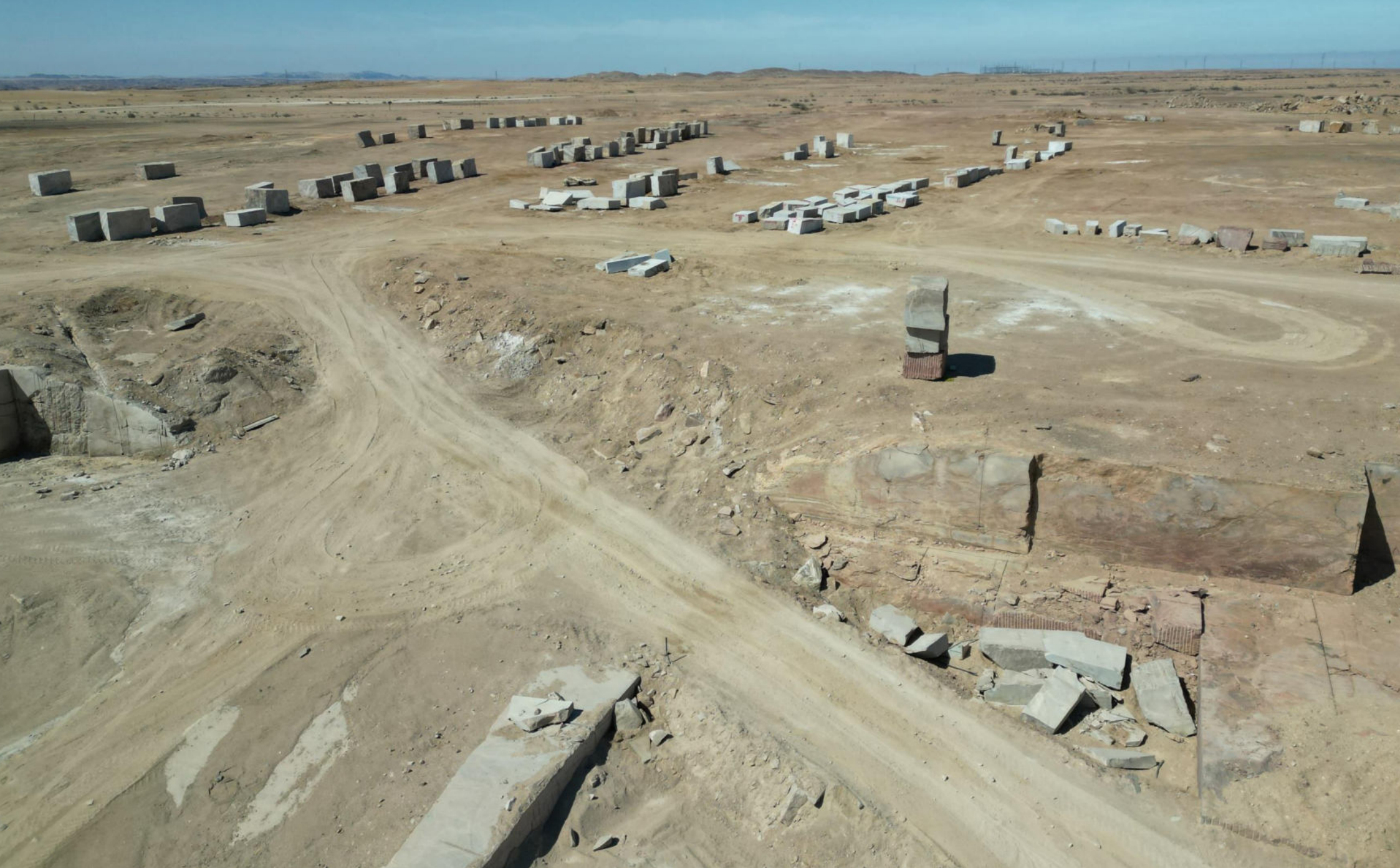
Plate 2.6: Extracted small 2 m x 1 m x 0,6 m (majority), and larger blocks 2,8 m x 1 ,3 x 0,8 m (minority) rectangular blocks stockpiled and sorted before being transported to the plant for final processing.
