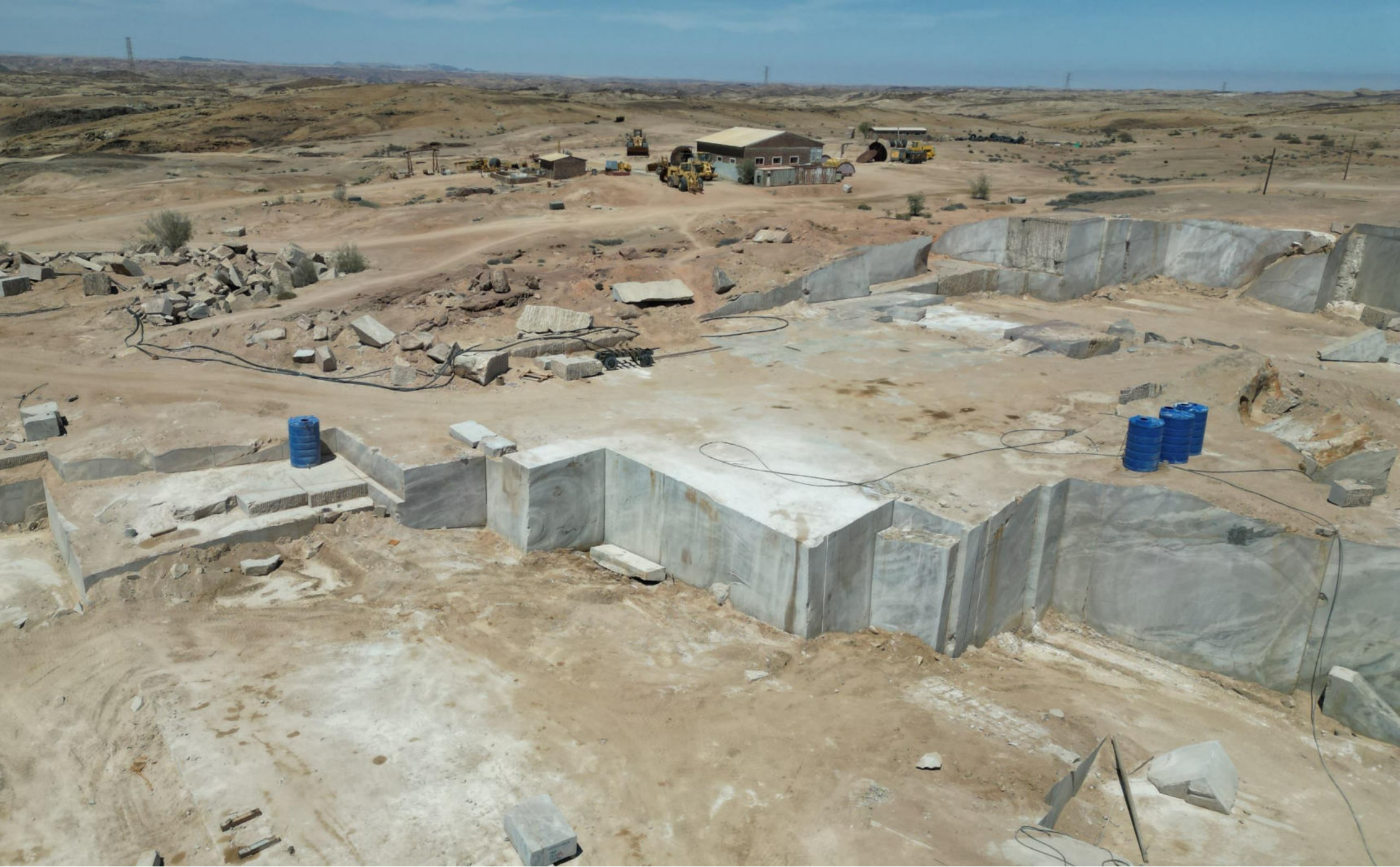
Plate 2.5: Drone image showing the south view of a working / extraction face at a granite quarry in the ML No. 123 with the workshop area in the background.
