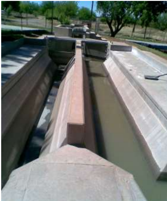
Figure 6: Proposed inlet works with grit removal channel
