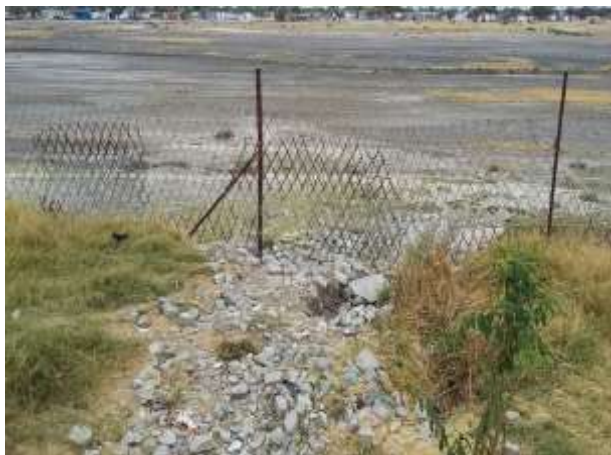
a) Soil erosion at the final pond outlet b) Area adjacent to final pond outlet - previous ponding Figure 3. Oshakati East Ponds – Final water health hazards at the ponds
