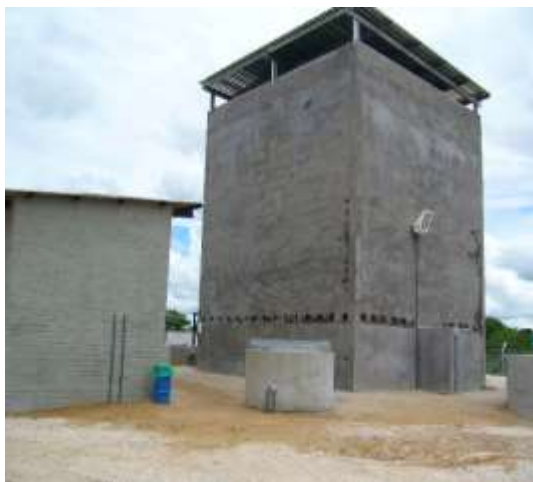
Figure 10a): Trickling filter tower
