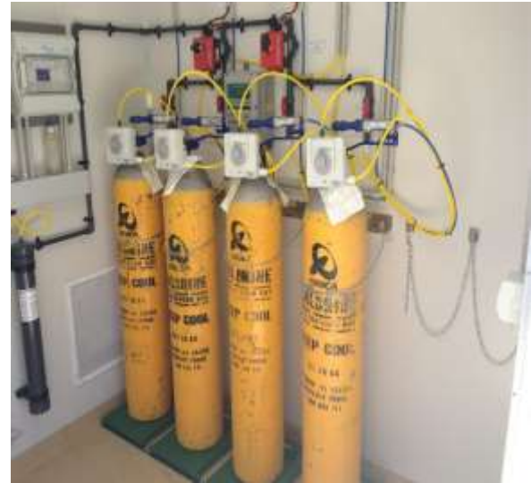
Figure 11: Typical medium-scale chlorine gas disinfection system (Hydramet)
