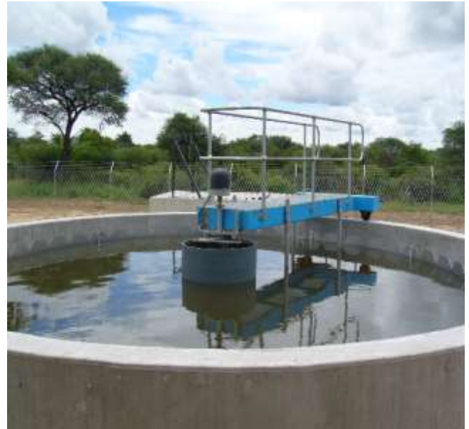
Figure 8. Clarifier with Rotating Bridge
