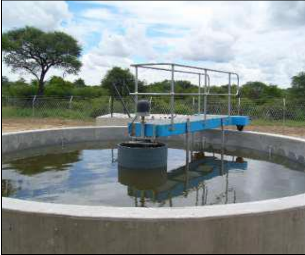
Figure 19: Clarifier with Rotating Bridge
