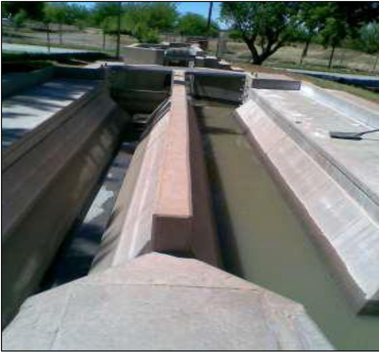
Figure 18: Proposed inlet works with grit removal channel
