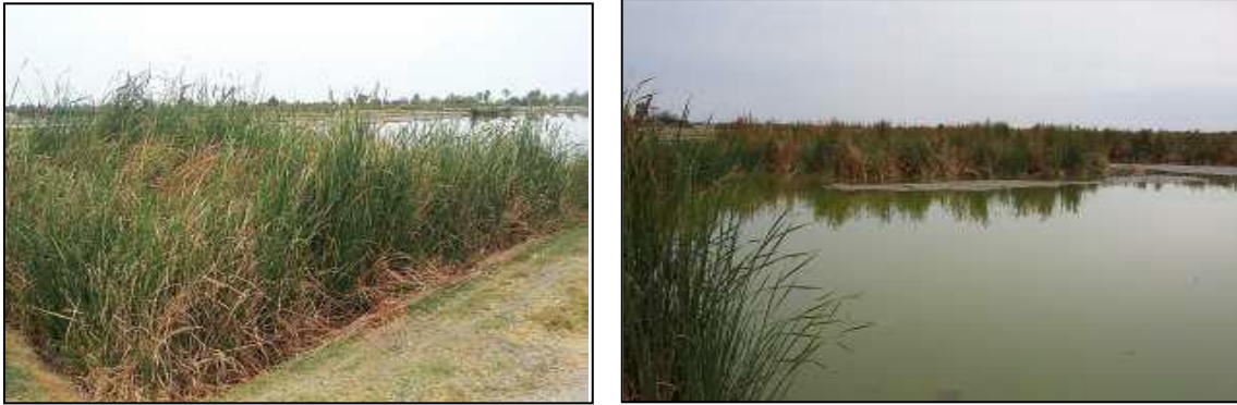
Figure 13: Oshakati East Ponds – Vegetation growth in primary and facultative ponds
