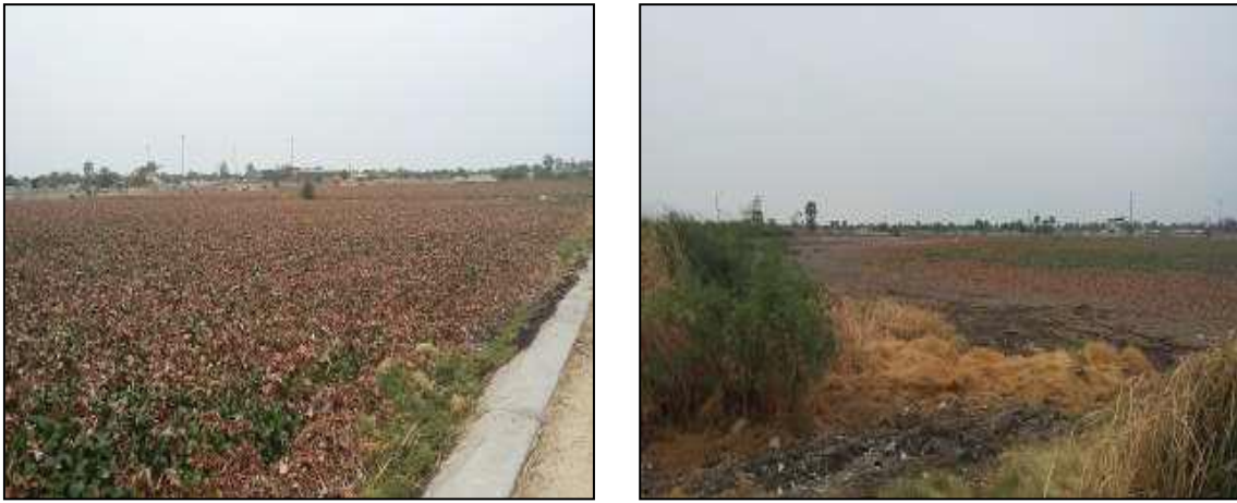
Figure 5: Oshakati West Ponds – Primary ponds overgrown
