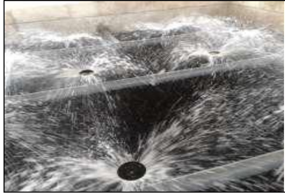
Figure 22: Trickling Tower with Wetting (Spray Nozzles) on Top
