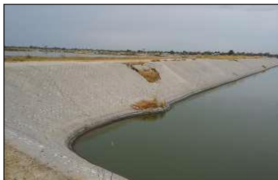
Figure 12: Oshakati East Ponds – Minor damage to embankments
