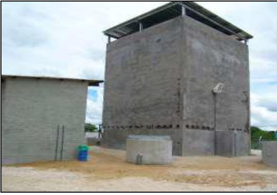
Figure 22: Trickling Tower with Wetting (Spray Nozzles) on Top
