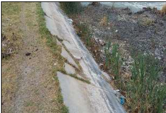
Figure 12: Oshakati East Ponds – Minor damage to embankments
