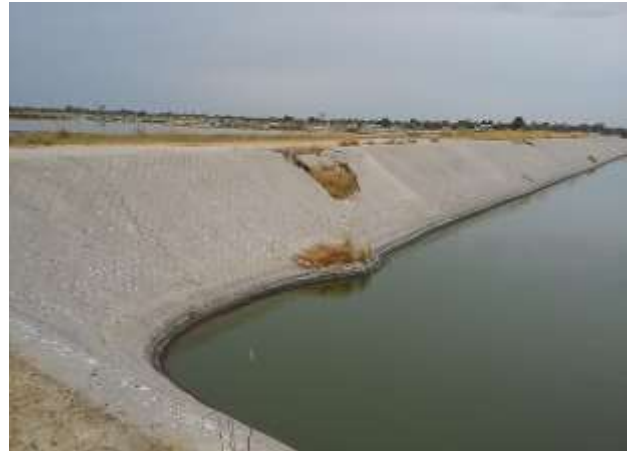
Figure 6. Oshakati East Ponds – Minor damage to embankments
