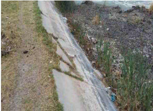
Figure 6. Oshakati East Ponds – Minor damage to embankments
