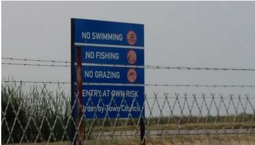
Figure 9. Oshakati West Ponds – damaged fence and evidence of fishing activities
