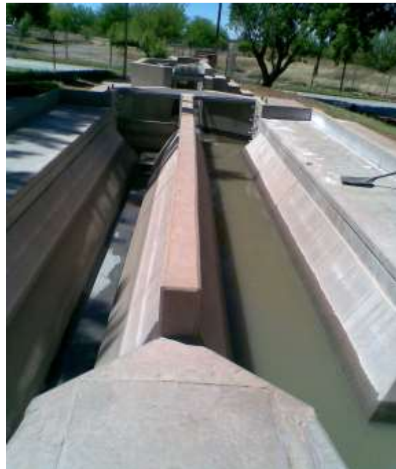
Figure C2: Proposed Inlet works with Grit Removal Channel
