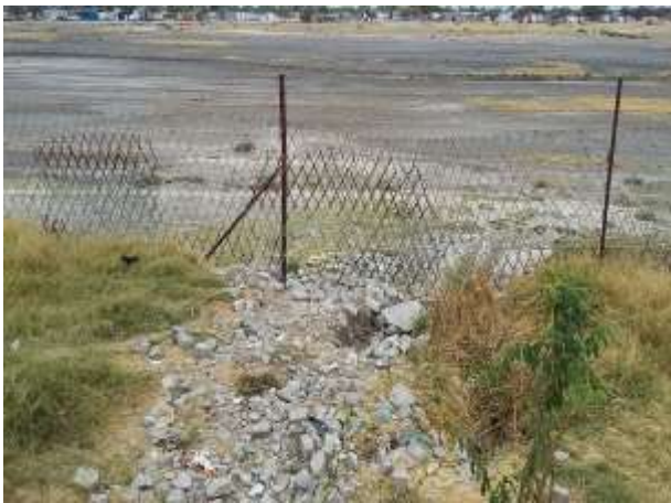
a) Soil erosion at the final pond outlet b) Area adjacent to final pond outlet - previous ponding Figure 8. Oshakati East Ponds – Final water health hazards at the ponds
