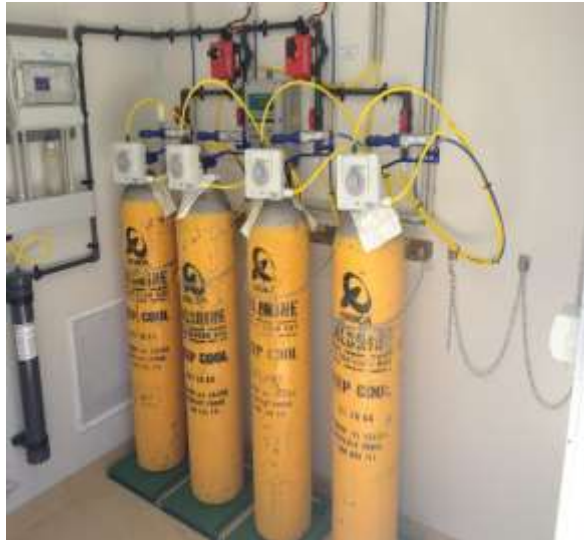
Figure C6: Typical medium-scale chlorine gas disinfection system (Hydramet)
