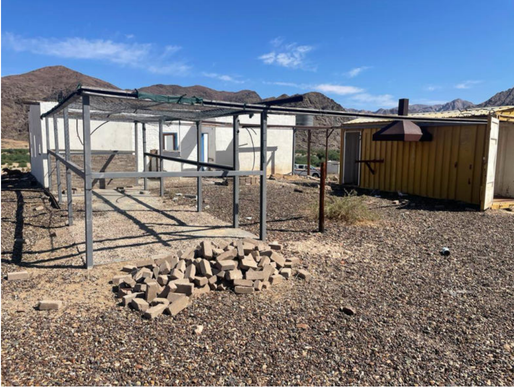
Figure 3: The remains of the residential house and storage container on ML 130. Source: Own photograph
