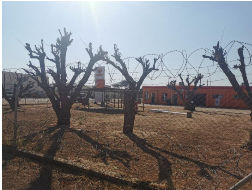
Figure 2-3: Site office building and Warehouse
