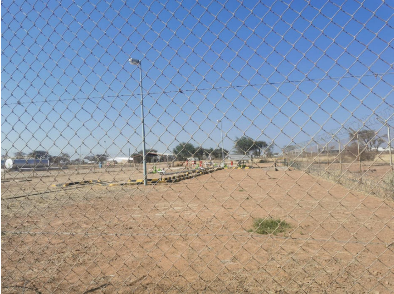
Figure 2-2: The rail siding located on the immediate southeastern side of the Depot
