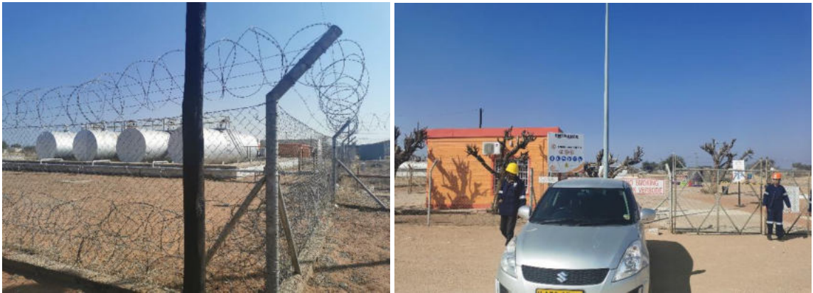
Figure 2-12: The mesh wire around the Depot site
