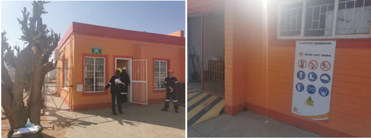
Figure 2-4: A closer view of the site office building and Warehouse
